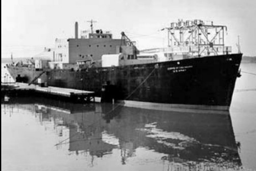
The MH-1A installed in "The Sturgis"
