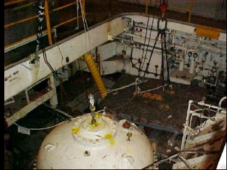
Containment vessel of the MH-1A reactor
